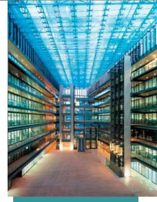
Spanish energy giant, Endesa, fills its Madrid headquarters atrium with daylight using an energy-efficient, ventilated glass roof made with DuPont™ SentryGlas®.
